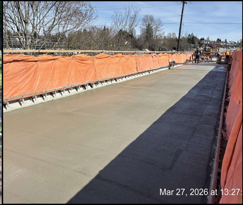
Figure 3: South bridge concrete placement
