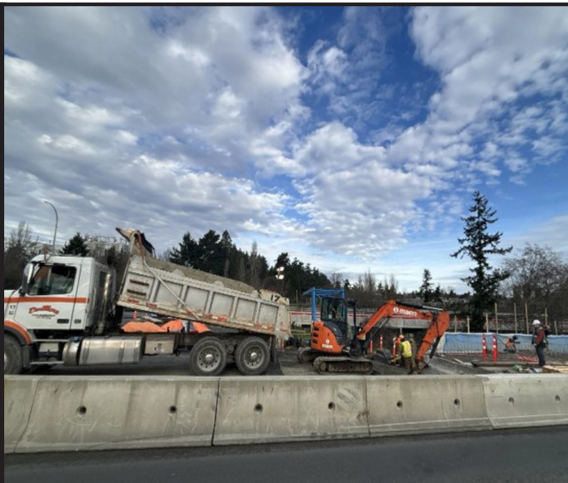
Figure 5: Bridge Excavation Fill (BEF) material placement and compaction at the west approach slab of the South Colquitz Bridge.
