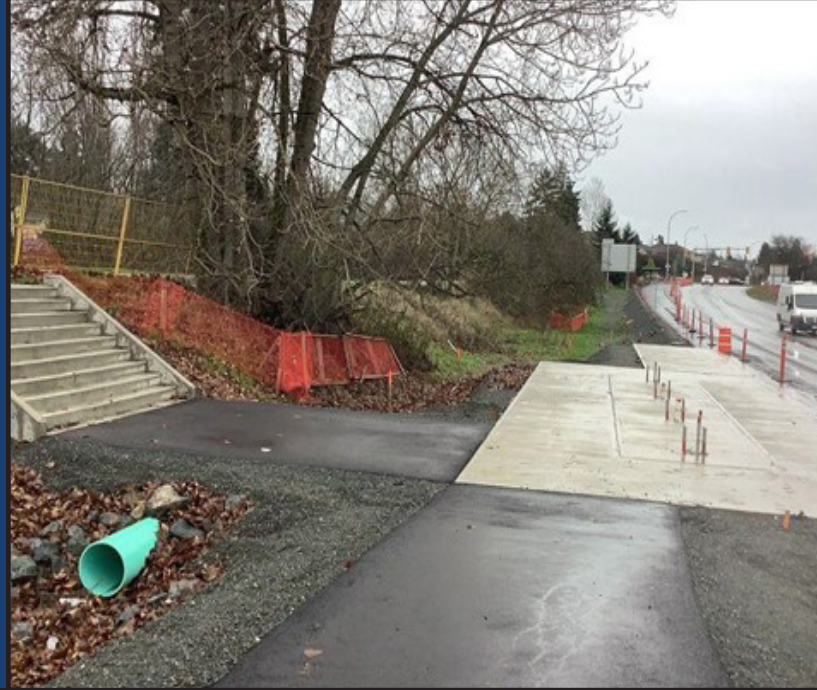
Figure 3: Completed access stairs connecting the Galloping Goose Regional Trail to the future bus stop area.
