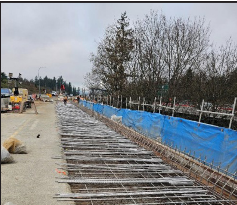
Figure 4: Crews installing rebar for the north deck extension of the South Colquitz Bridge.
