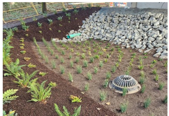
Figure 1: Rain garden completed below the South Colquitz Bridge to support stormwater management.
