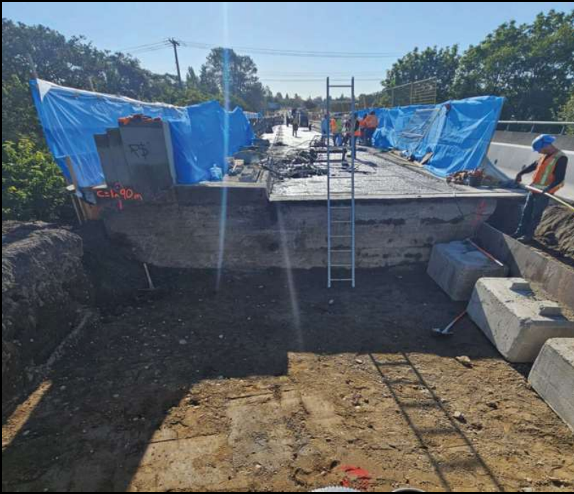
Figure 2: North Bridge West Abutment Excavation
