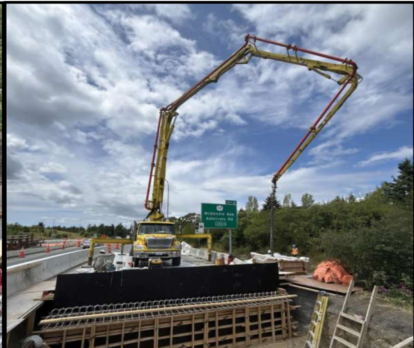
Figure 5: North Bridge Concrete Pour
