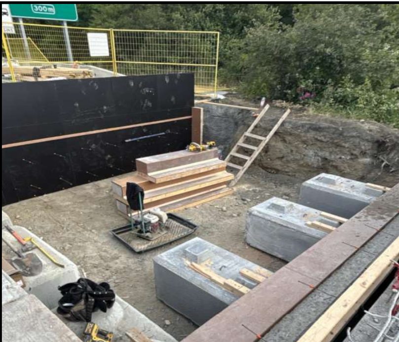
Figure 4: North Bridge Formwork Installation
