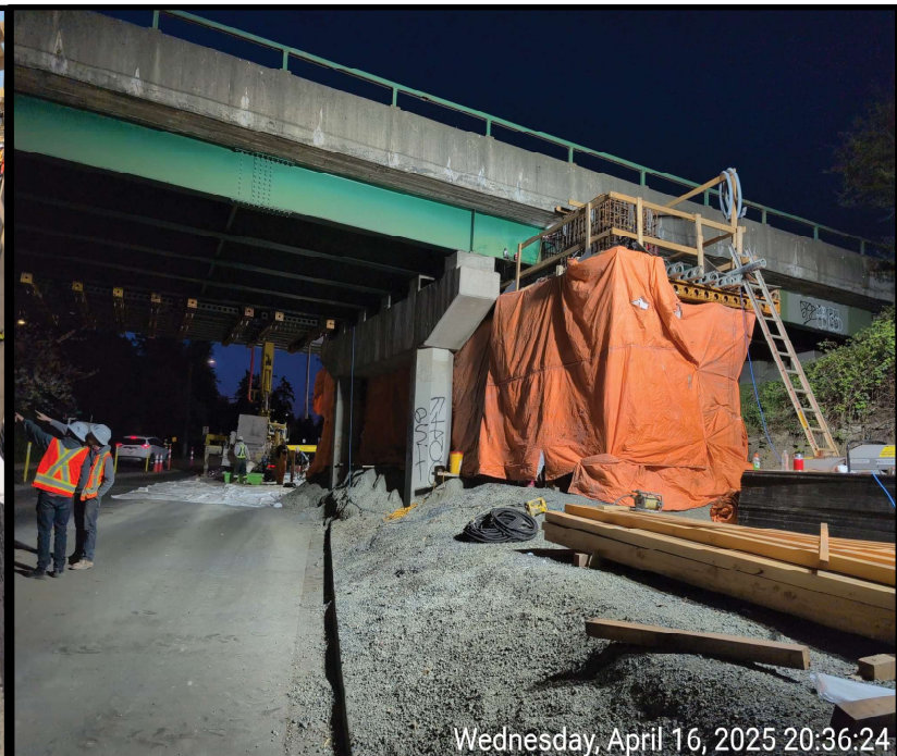
Figure 5: Heating and Hoarding for Concrete Curing
