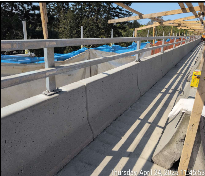
Figure 4: Installation of South Bridge Railing
