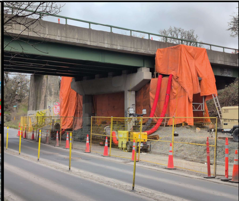
Figure 5: Heating and Hoarding for Concrete Curing
