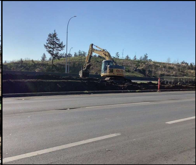
Figure 3: Works Along West Median on Highway 1
