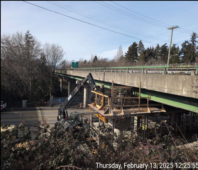
Figure 2: Work Along North Bridge Bent
