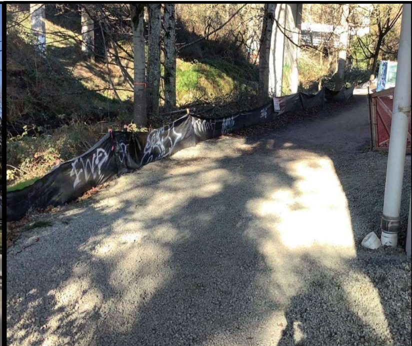
Figure 5: Silt Fencing Along Multi-Use Path
