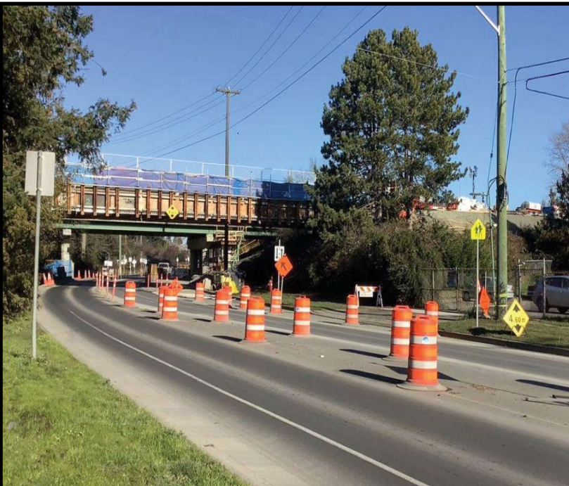
Figure 4: Traffic Management Along Burnside Road
